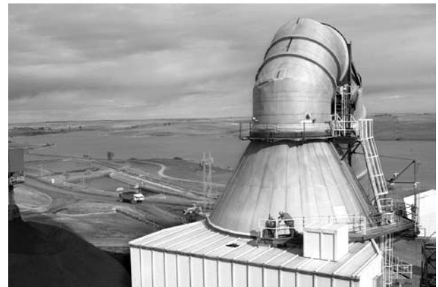
As part of the Minnkota settlement agreement, the Young 2 sulfur dioxide scrubber will be modified in 2010 to increase its removal efficiency. A new scrubber will be constructed for Young 1 in 2011.
