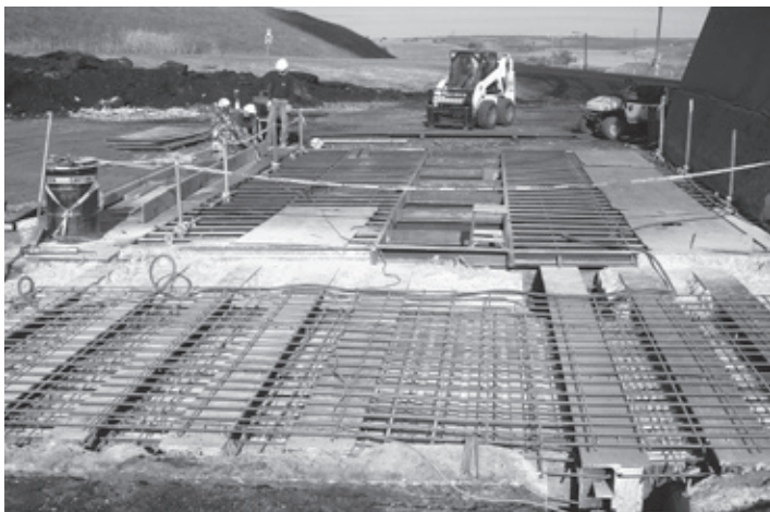
The Young 2 coal receiving area was modified to include a strengthened metal grating system to handle larger coal trucks.
